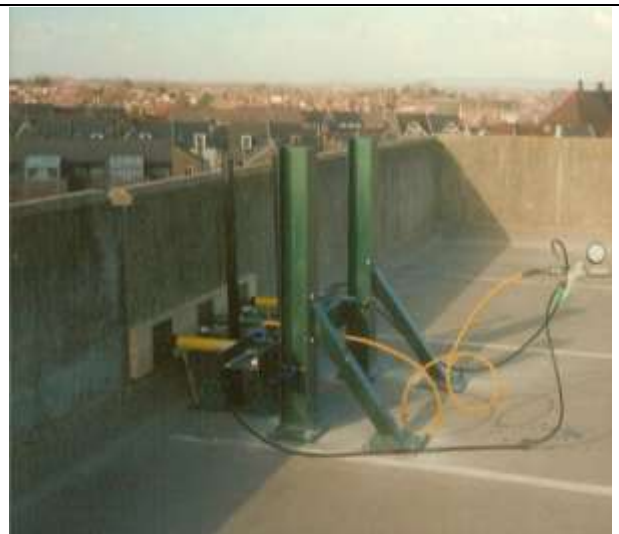
Testing of Car park parapet panel
