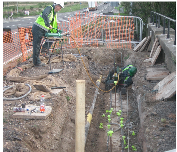
Tensile testing of insitu deformed rebar
